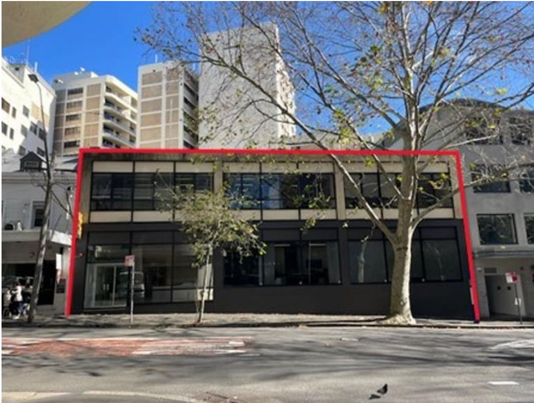
Figure 2: 47-51 Riley Street, Woolloomooloo, viewed from Riley Street and outlined in red
